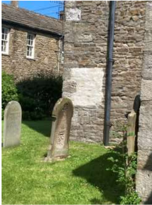
Test patches on south wall
